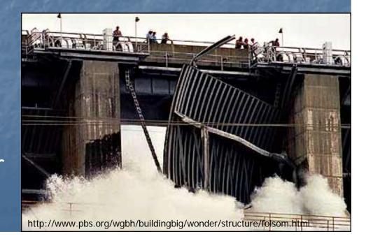
5 radial gates for flood control are 13m wide 15.2m high 3 radial emergency gates are 13m wide and 16.2m high Cause of Failure: **Trunnion** friction moment was the key factor, and was omitted in original design calculation
