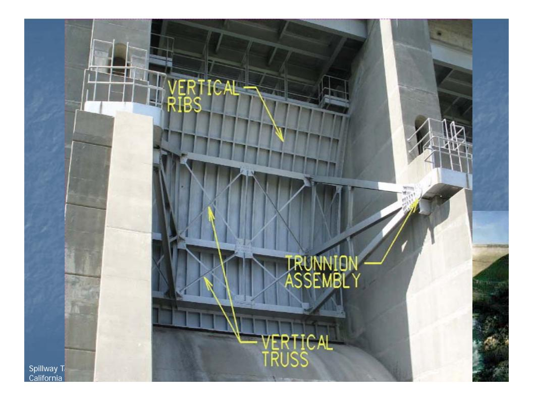
So what is trunnion friction moment: the product of the friction force and the pin radius
